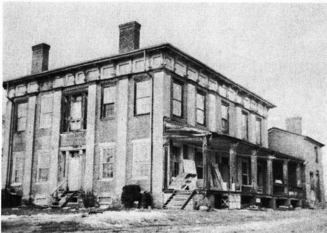
Figure III-25. Rear veranda prior to Fairfax' 1954 renovation.
