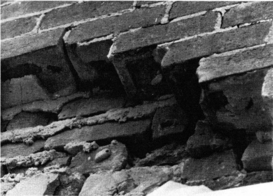
Figure III-66. Frogged bricks used in the construction of Fairfax.
