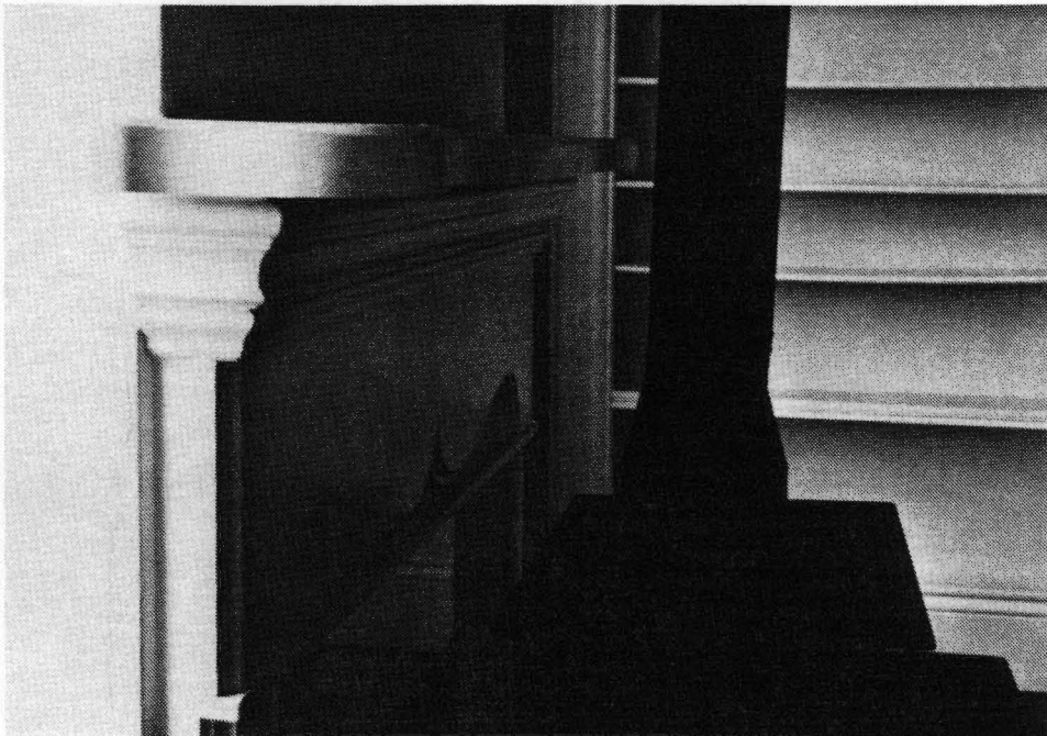
Figure III-44. Corresponding mantle shelf with Grecian moldings.
