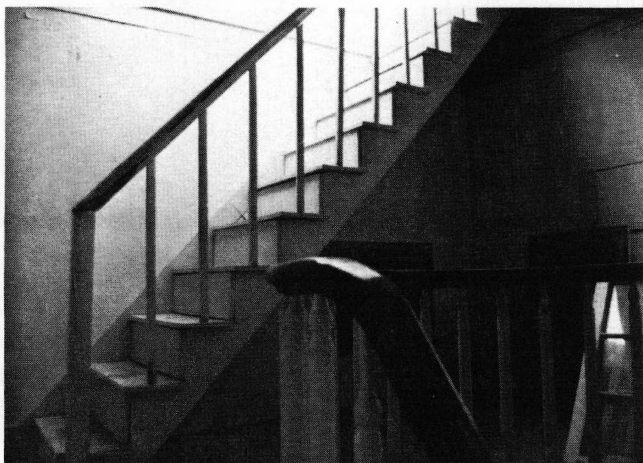
Figure III-71. Stairway leading to Fairfax' roof deck.
