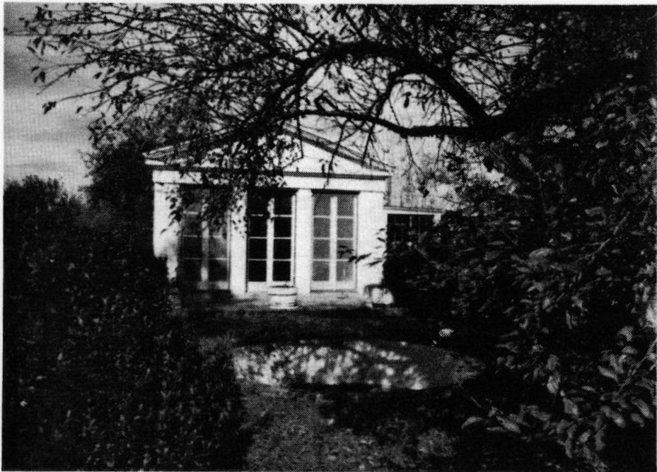
Figure III-24. South facade of guest house.
