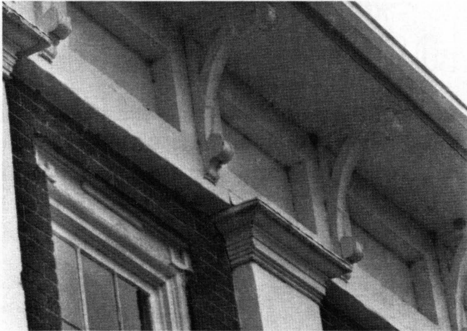
Figure III-14. Frieze, brackets and overhanging eaves at Fairfax.
