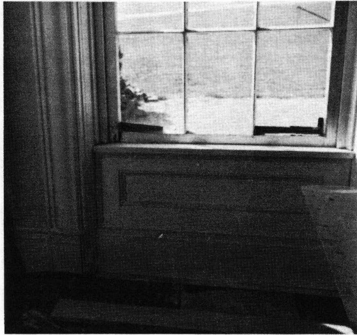
Figure III-41. Pine panel between sill and base molding at Fairfax.
