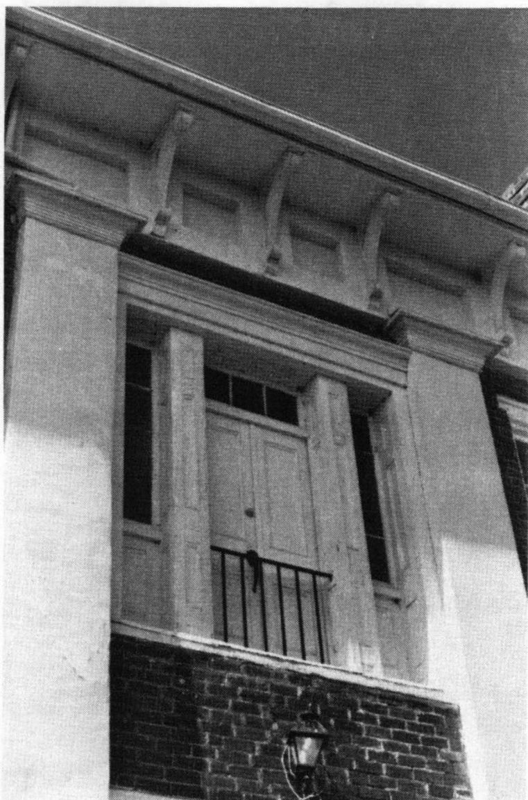
Figure II-1. Pilaster and frieze features on Fairfax' south facade.
